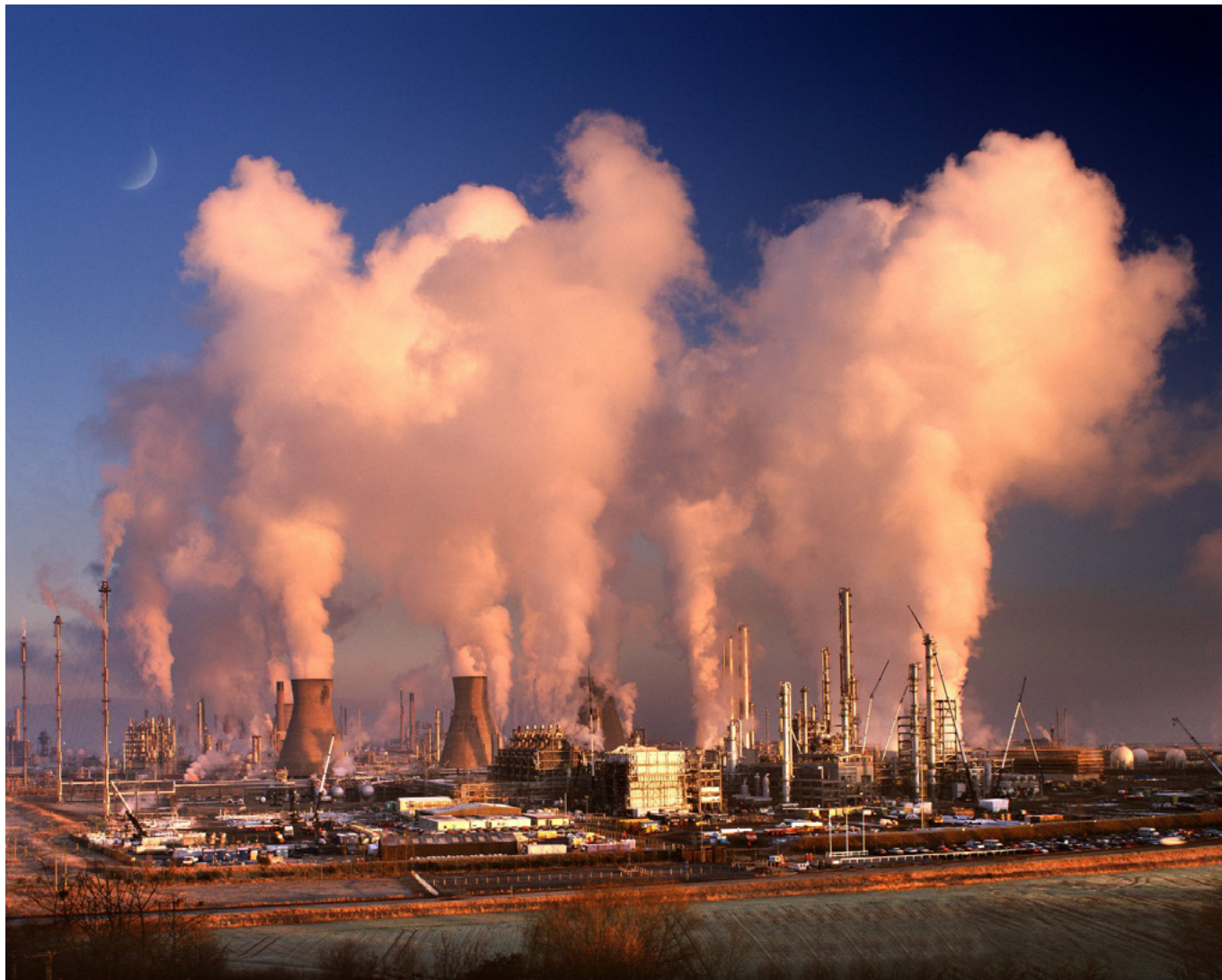
Grangemouth Petro Chemical Plant
